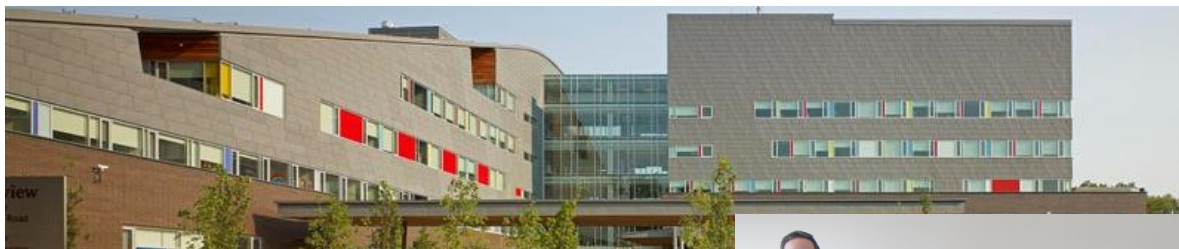
Holland Bloorview Kids Rehabilitation Hospital, Toronto
